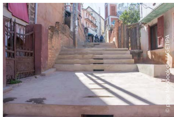
Image 34 : Construction of a staircase.
